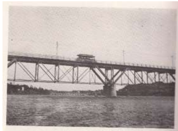
Fig. 3: 1902-1942 Trolley Bridge, looking (1920c.) east to the Erie Canal Aqueduct. 4
