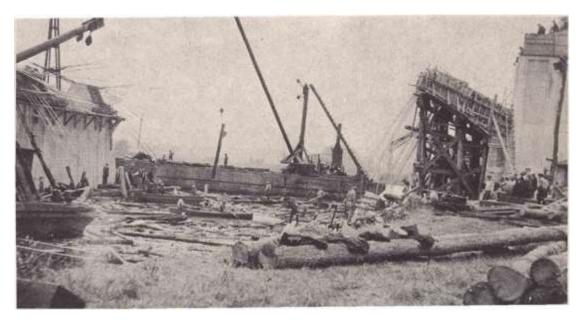
Fig. 5: Western Gateway Bridge Construction Collapse at Scotia to Hog Island Crossing 1923<sup>iii</sup>
